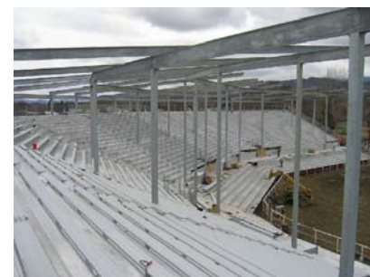
Omak Stampede grounds during construction- Photo by Chad Short
